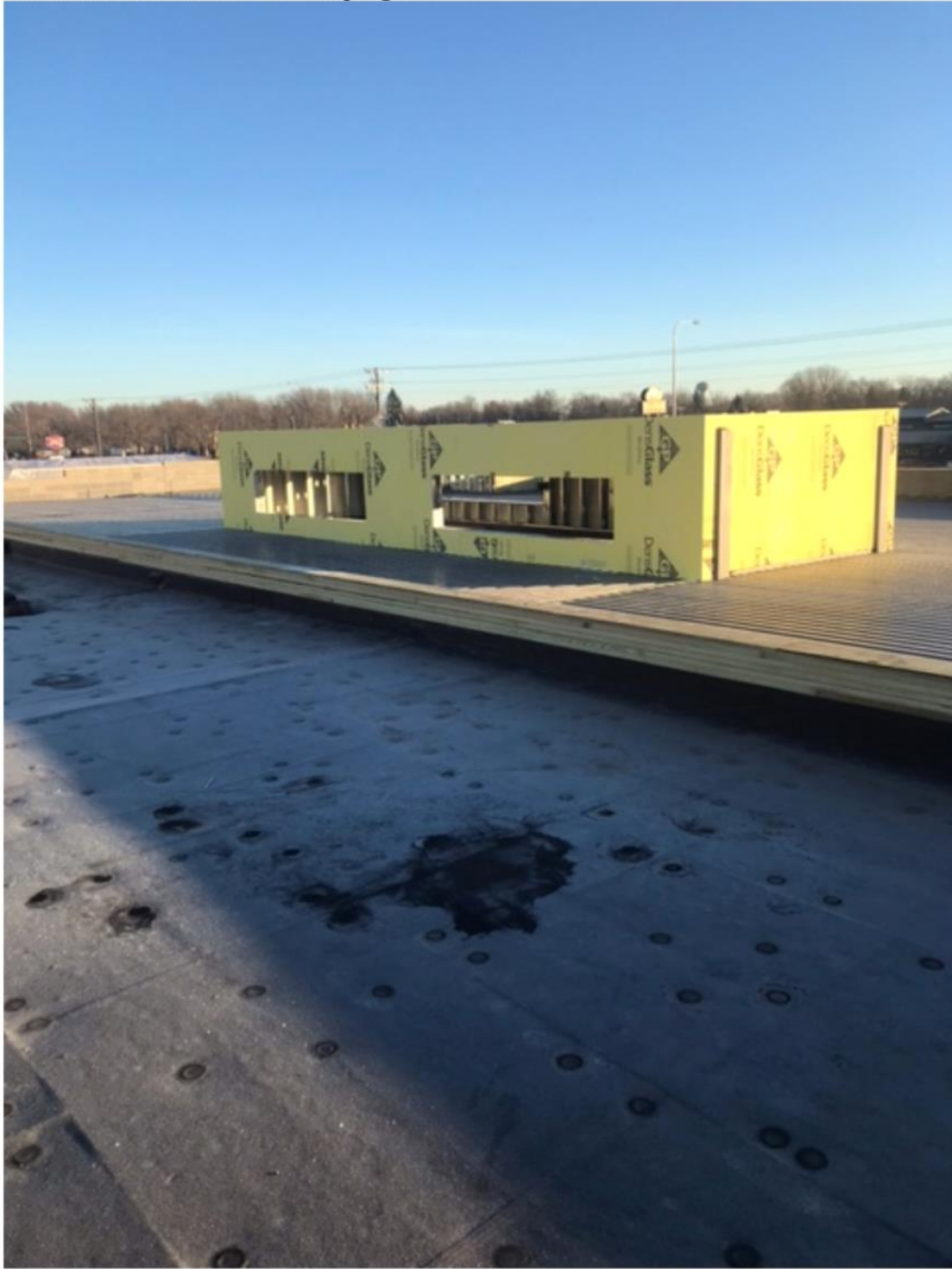
“Area A Roof Construction” In-progress
