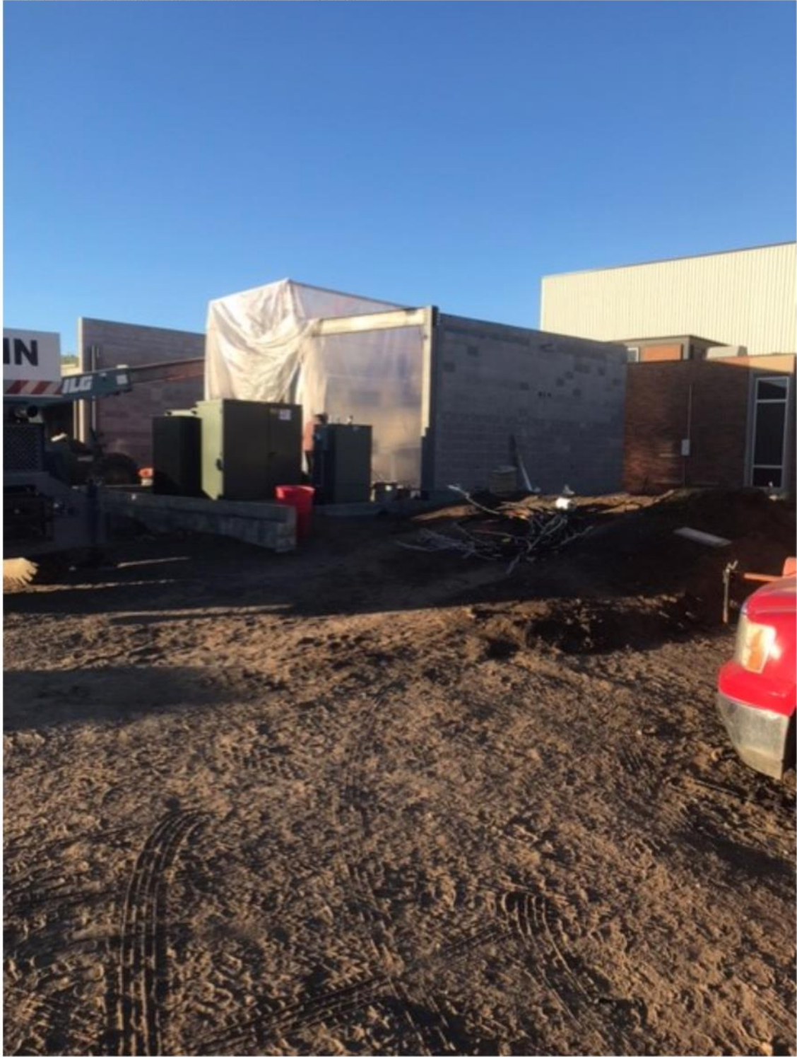
“Area B Masonry Construction” In-progress
