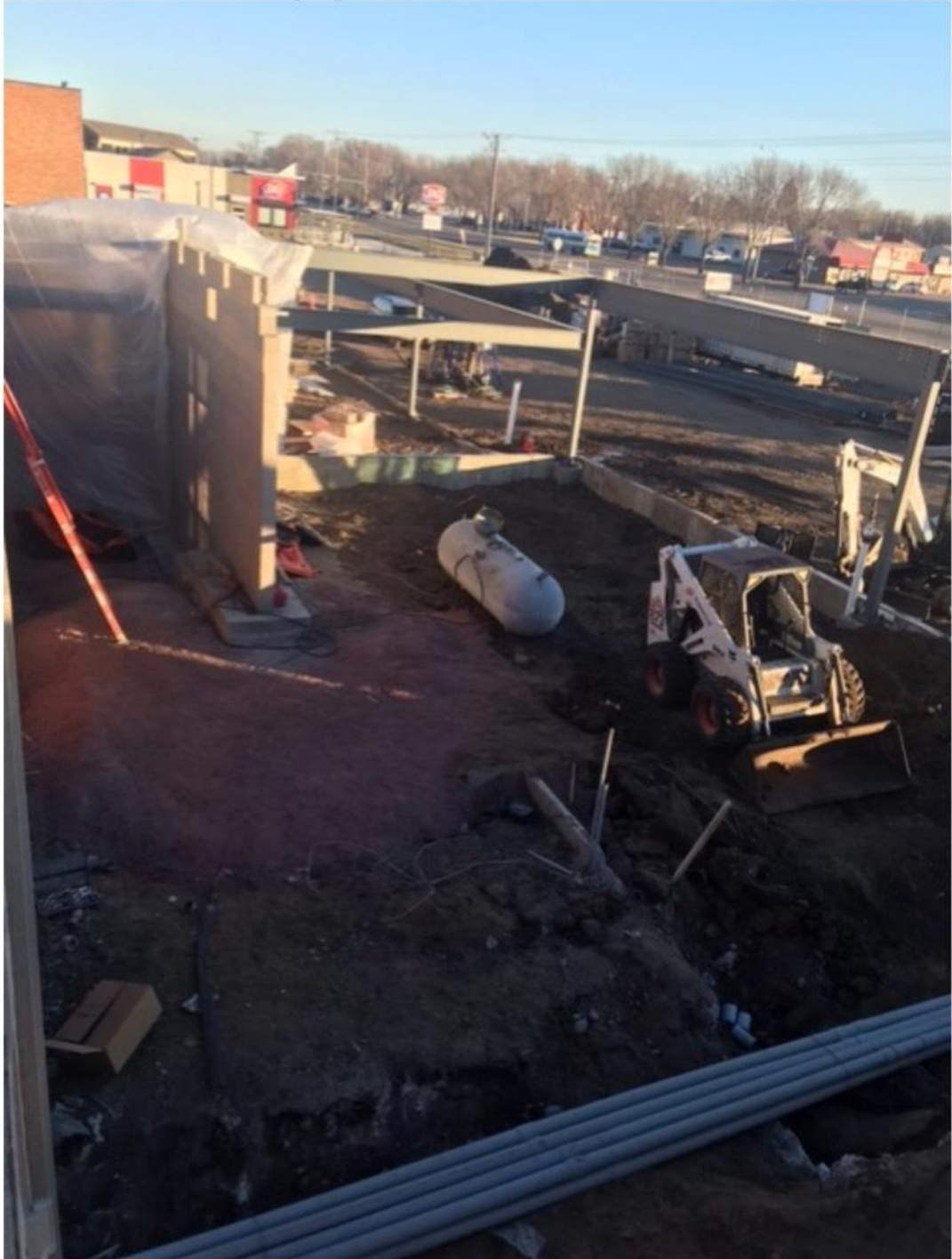
“Area B Construction” In-progress
