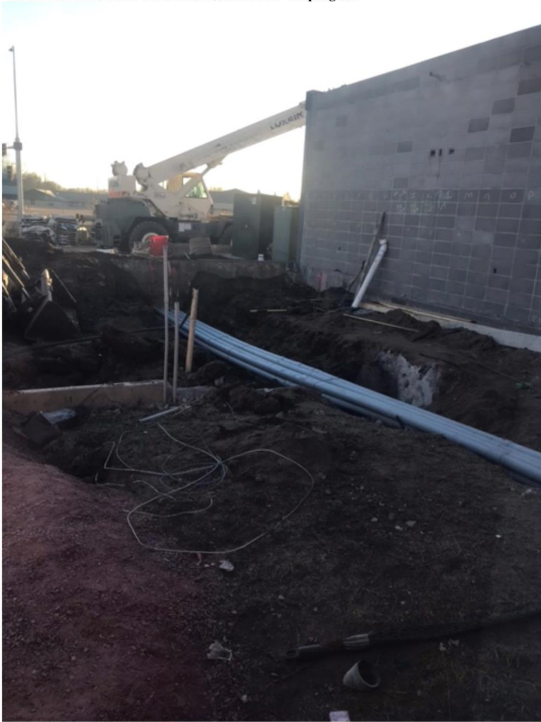
“Area B Transformer / Electrical Construction” In-progress
