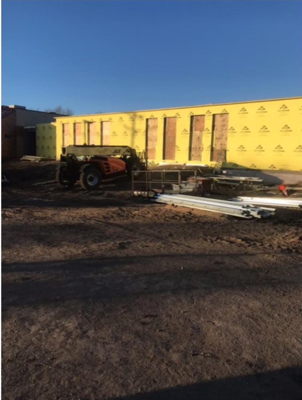
“Area A Enclosed & Construction In-progress”
