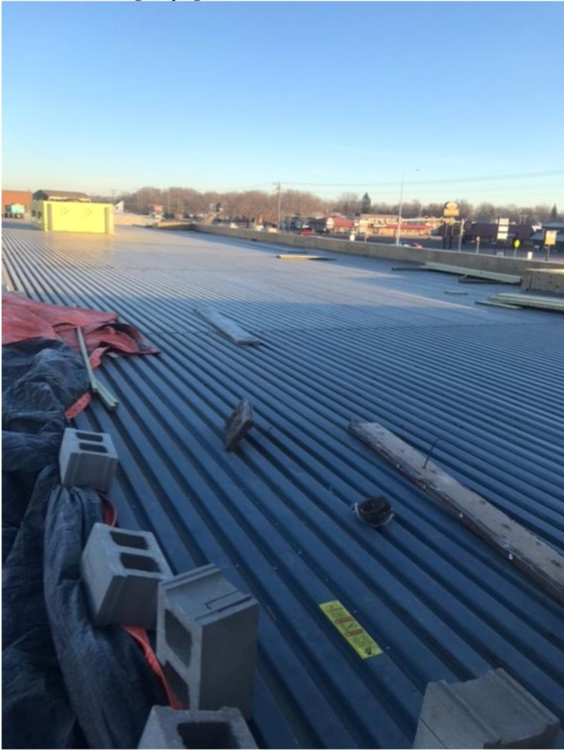
“Area A Roof Decking” In-progress
