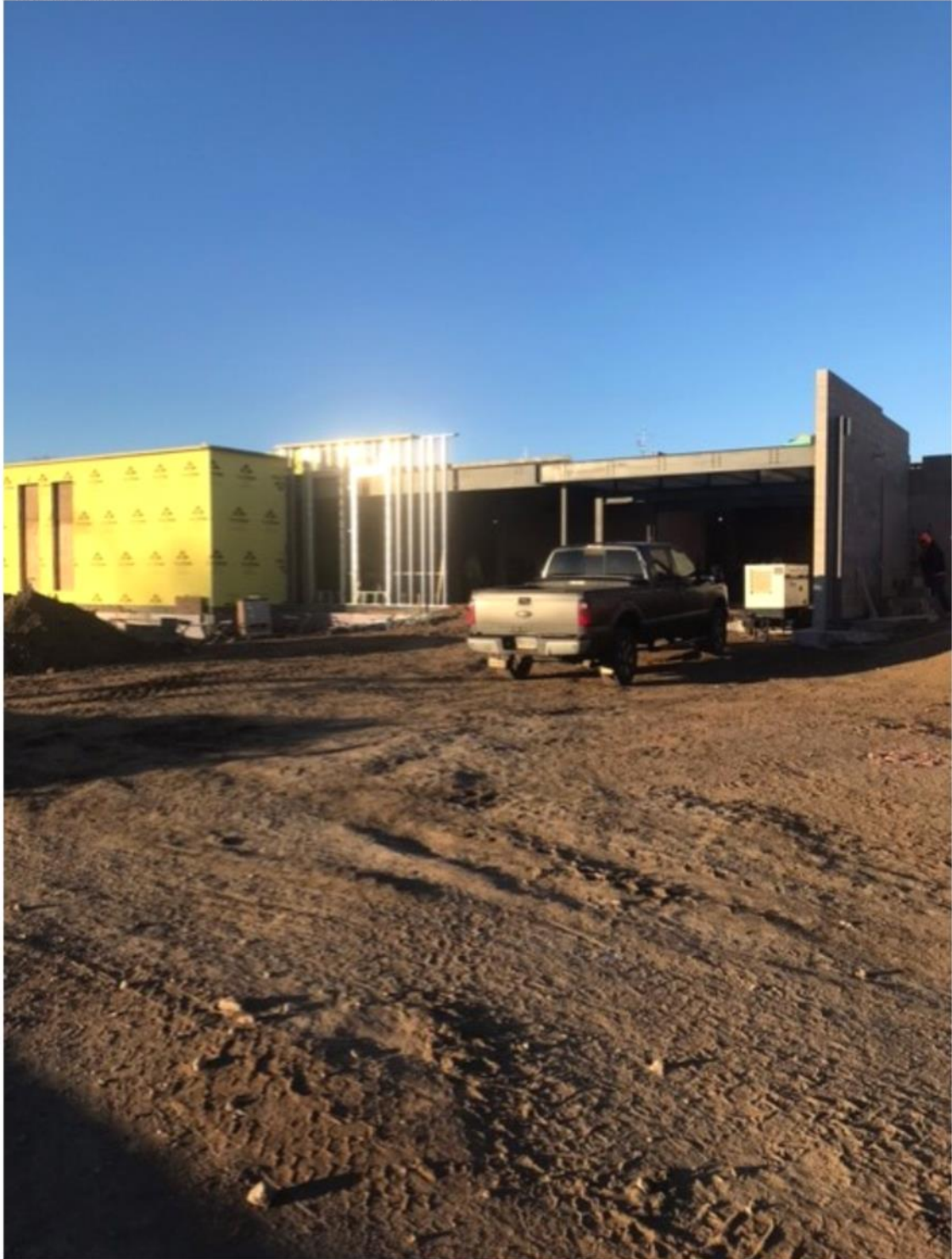
“Area A Steel Stud Construction” In-progress
