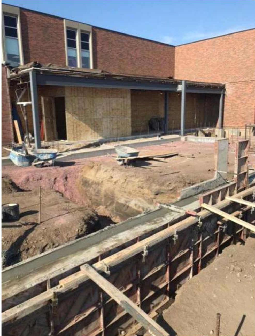
“Area B Entrance Structural Steel / Foundation Wall Construction” In-progress
