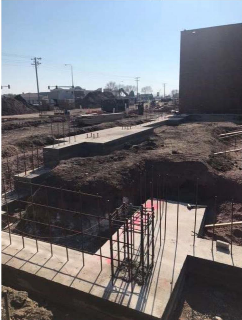
“Area C Footing / Foundation Wall Construction” In-progress
