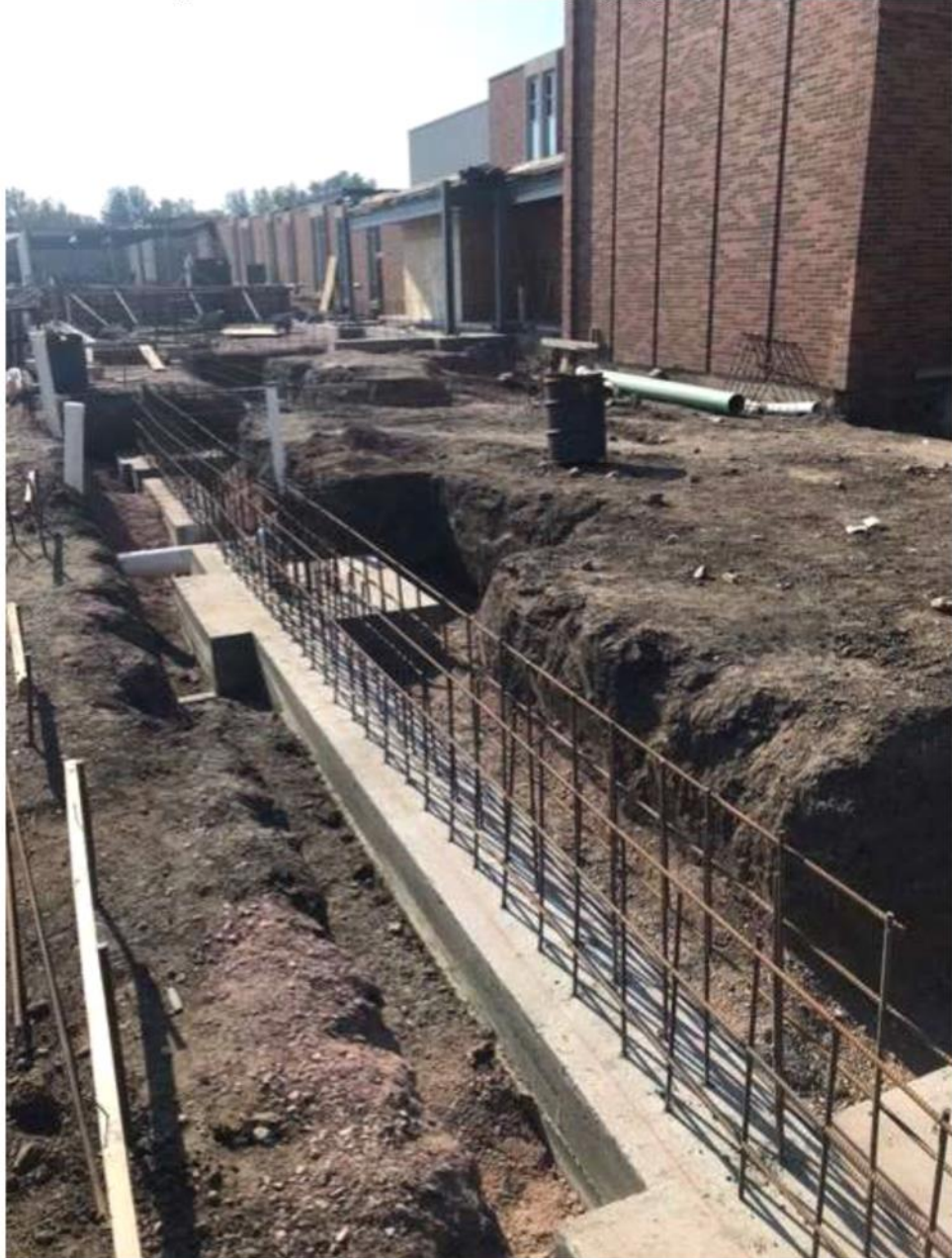
“Area C Footing / Foundation Wall Construction” In-progress
