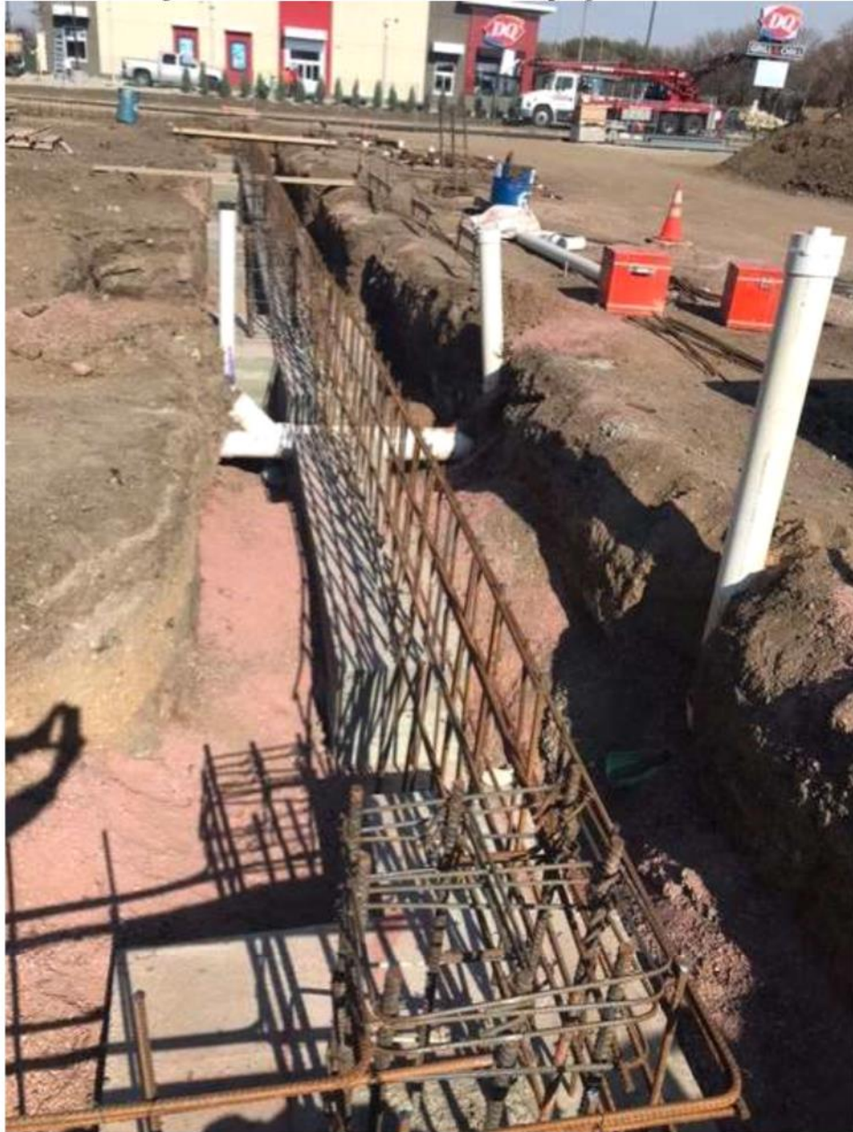
“Area C Footing / Foundation Wall Construction” In-progress
