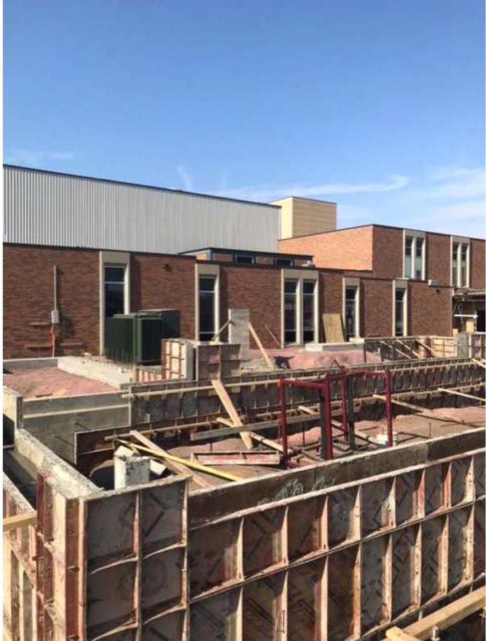
“Area B Foundation Wall Construction” In-progress
