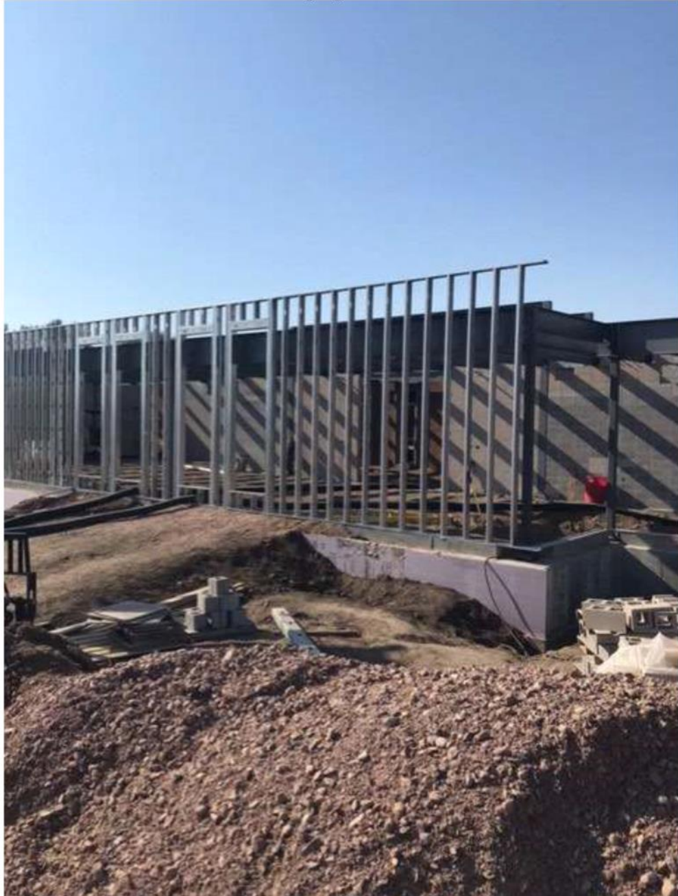
“Area A Steel Stud Construction” – In-progress
