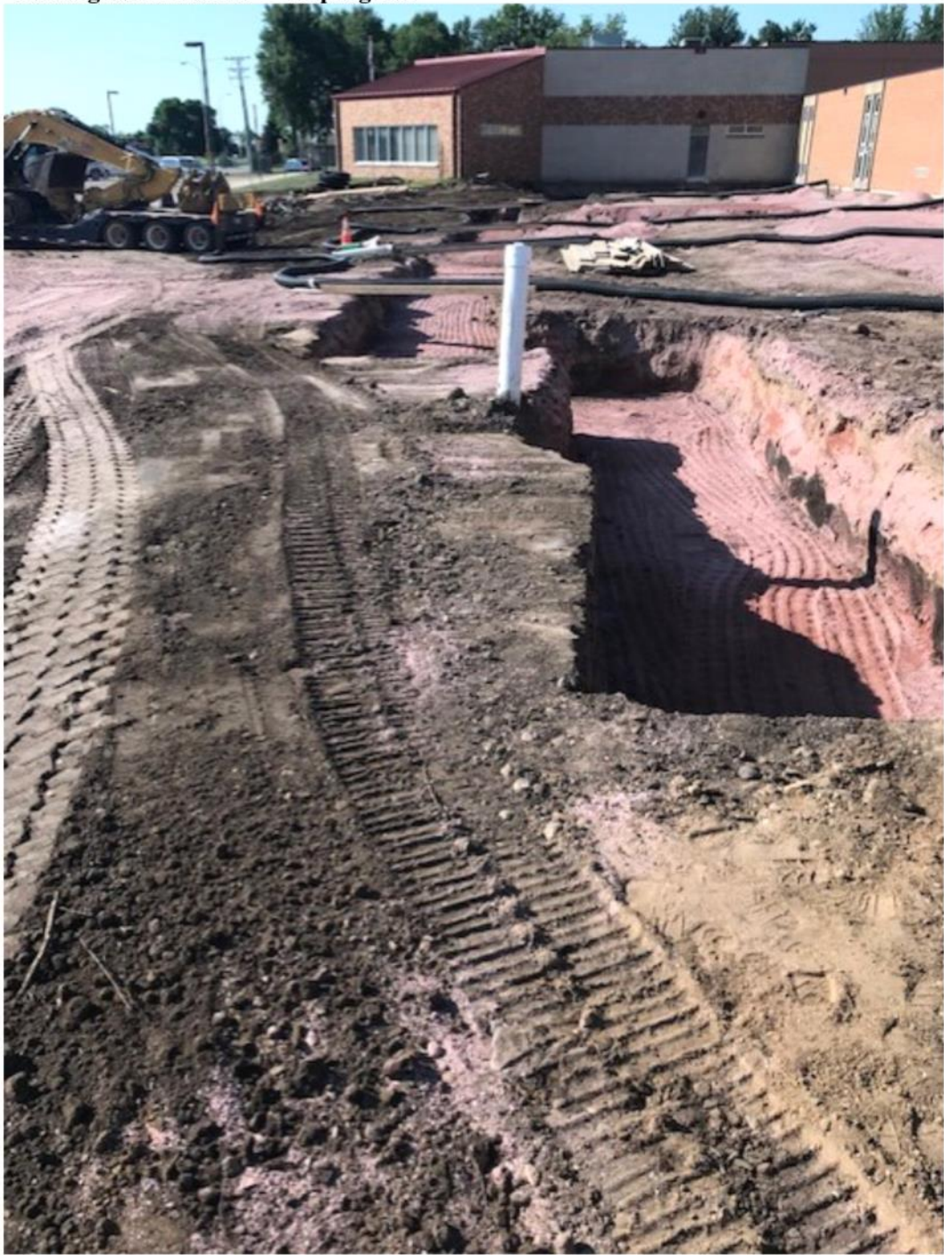
“Footing Construction” – In-progress
