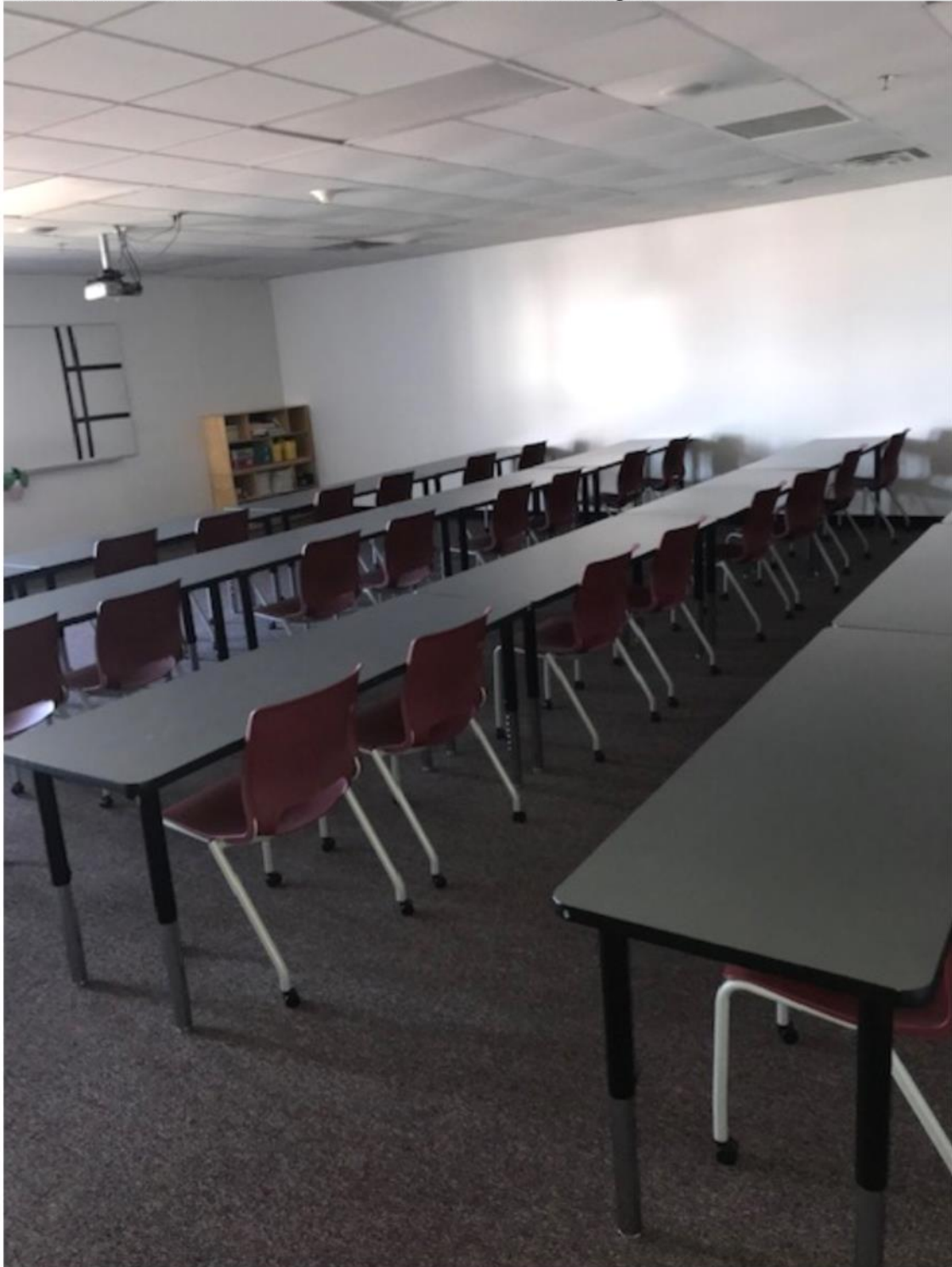
“Room 104 – B. Olson Classroom” Wall Construction Complete
