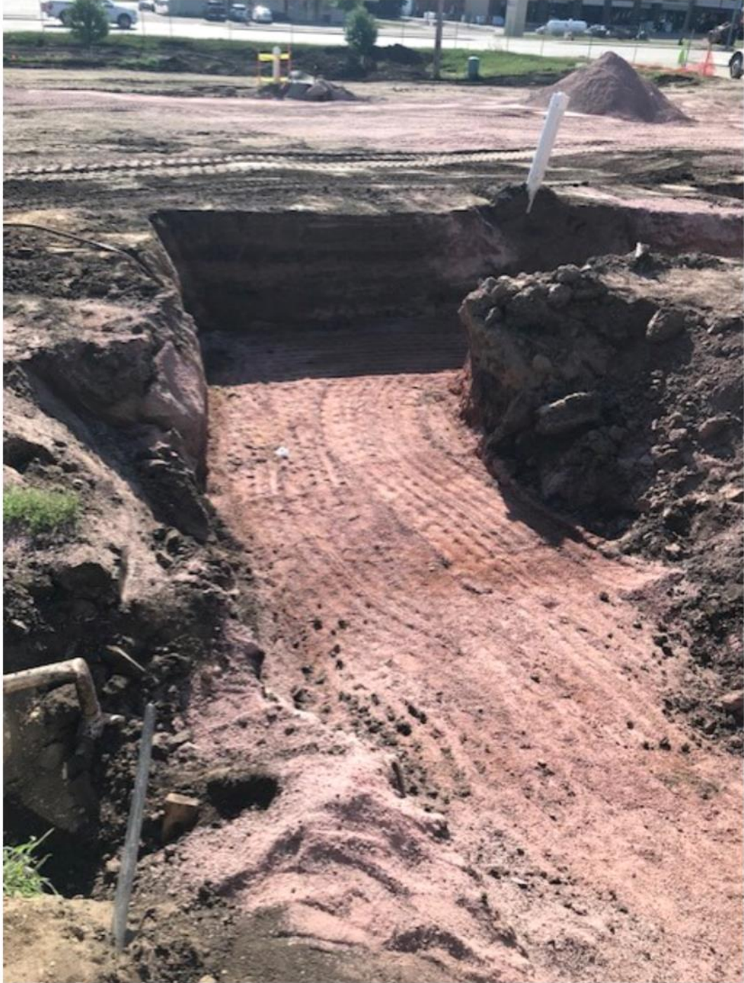
“Footing Construction” In-progress
