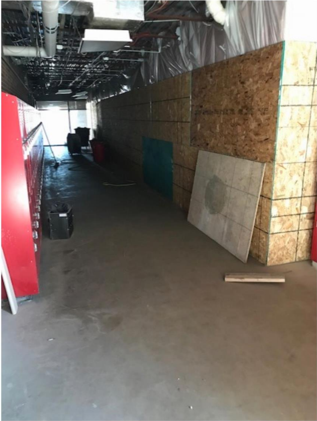
“Temporary Construction Wall” Hallway
