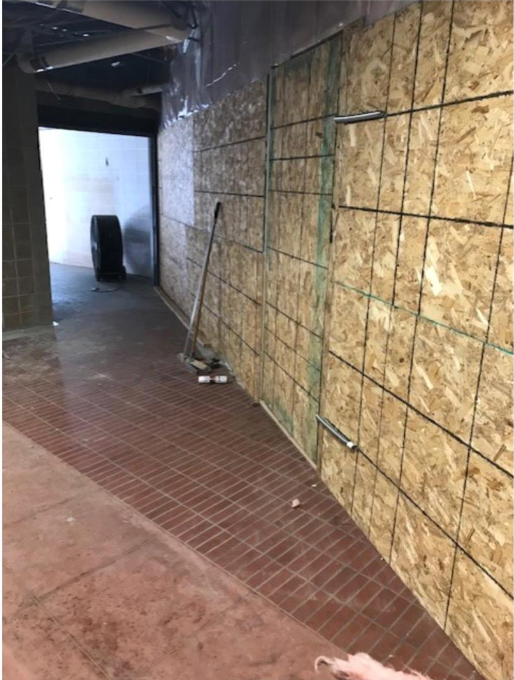
“Temporary Construction Wall” – East Exit / Ramped Hallway
