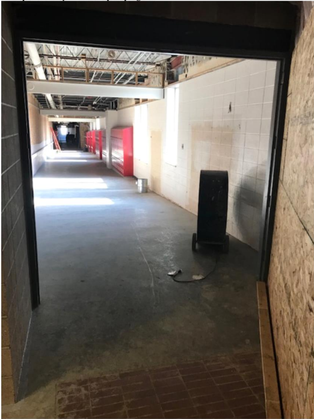
“Ramped Hallway” – Clean-up In-progress
