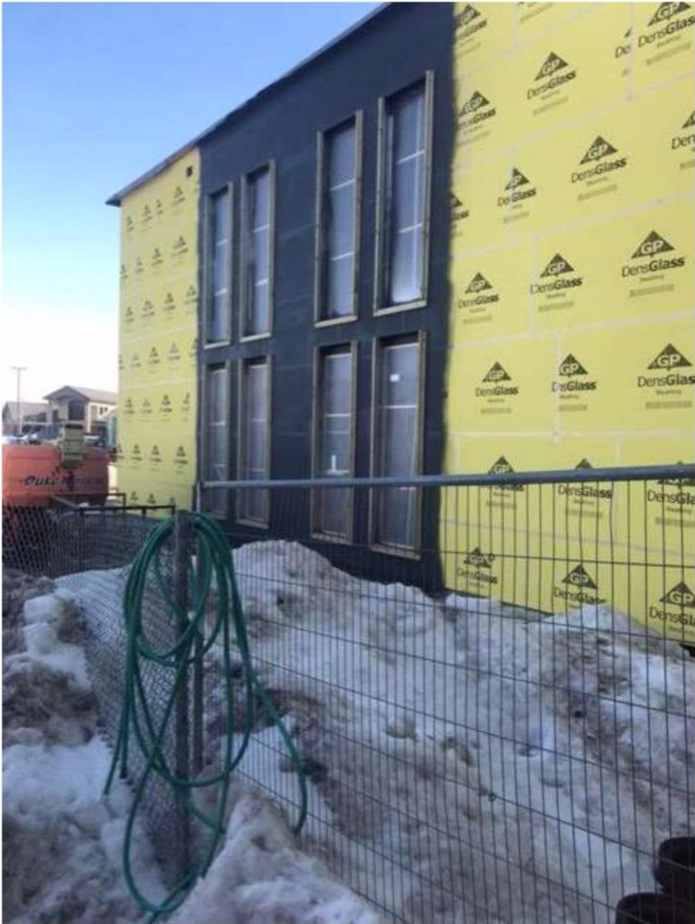
Area C – Precast Panel / Masonry In-progress
