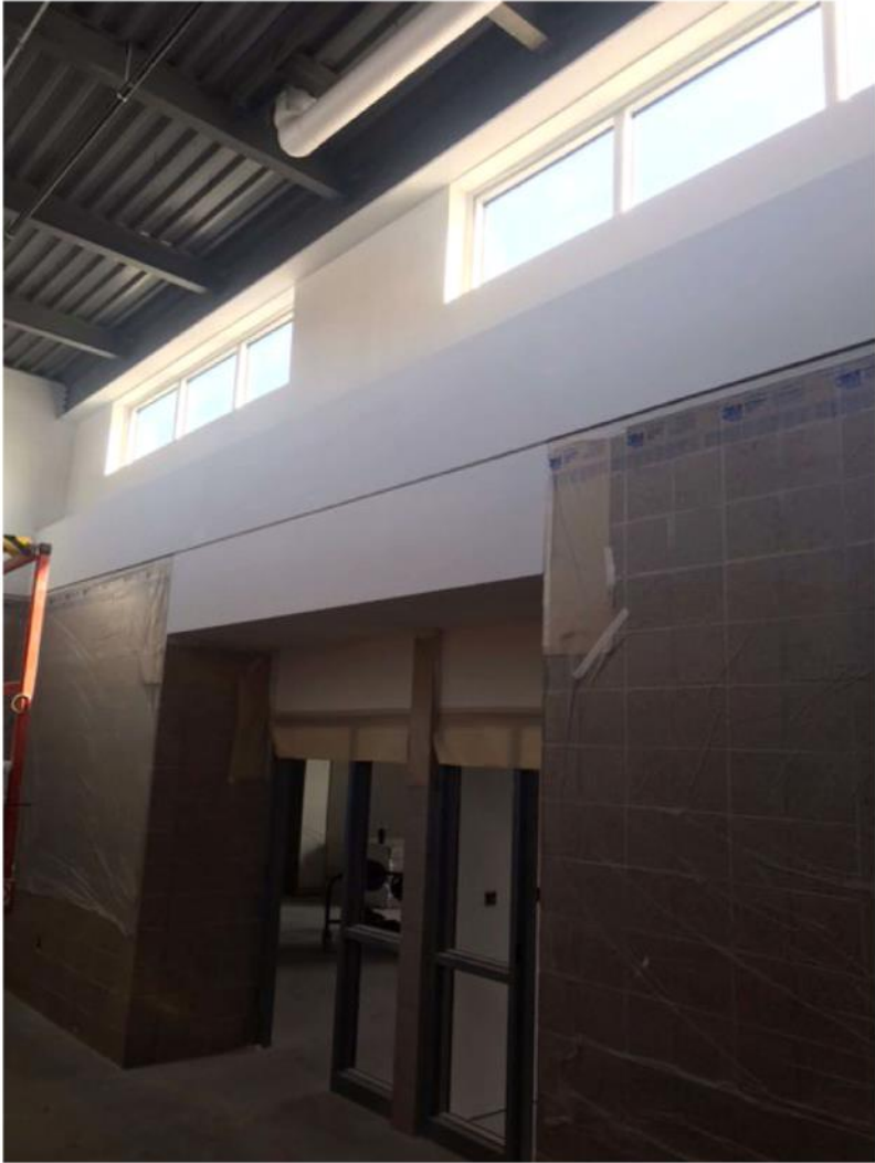
Area A Clearstory - Painting In-progress
