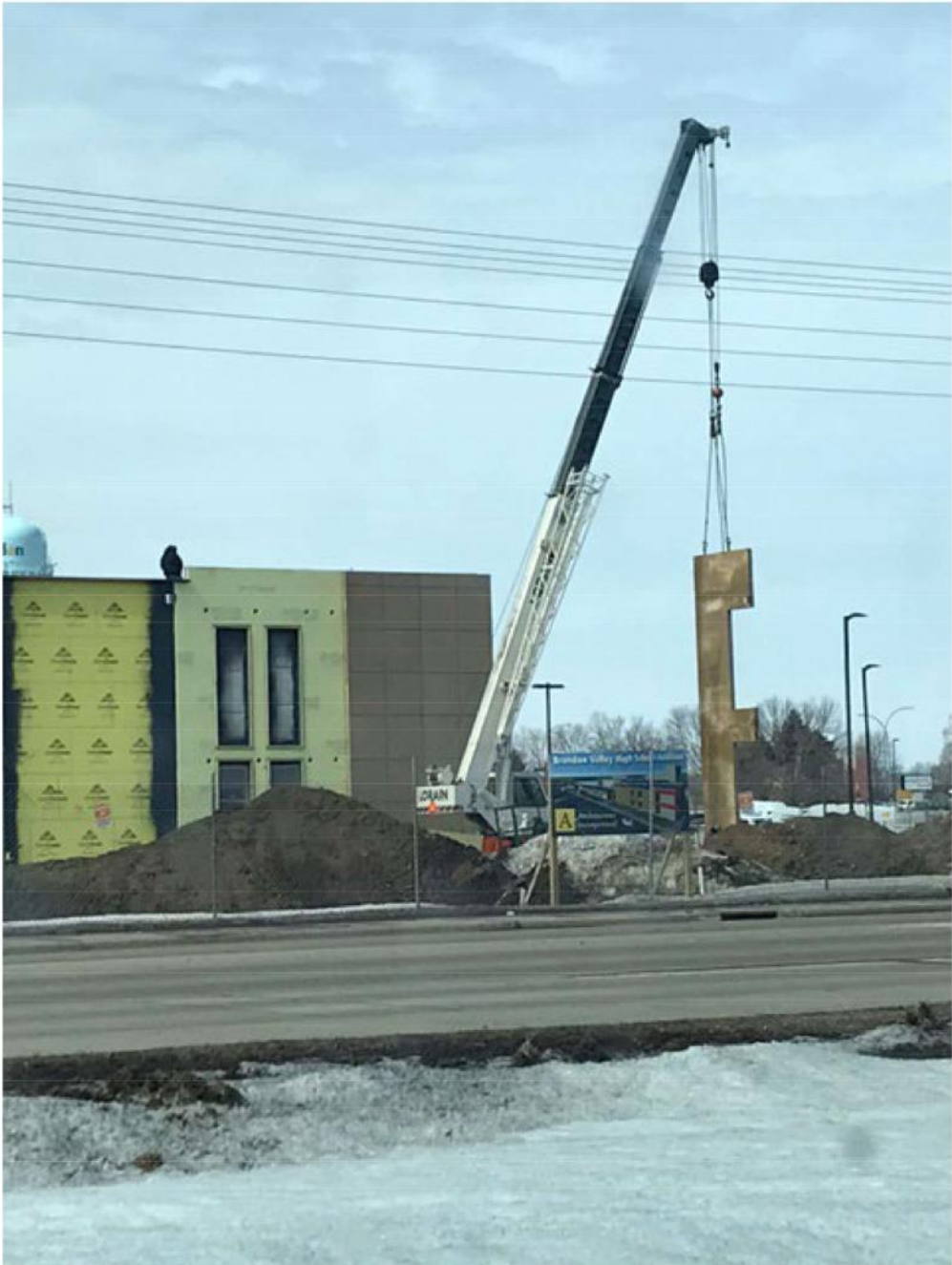
Area C – Precast Panel / Masonry In-progress
