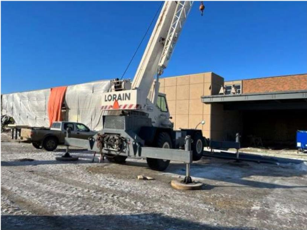
Area B (facing southwest) – Exterior Masonry Construction In-progress
